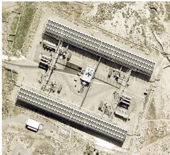
Aerial view of Steamboat Springs Geothermal Plant in Montana.
