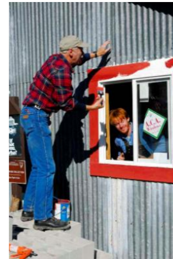
Volunteers installing a window at National Public Lands Day 2007
